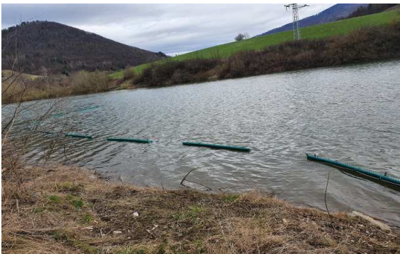
Figure 3. Installed floating trash barriers in the area of the Ružín water reservoir Source: authors (2023)
