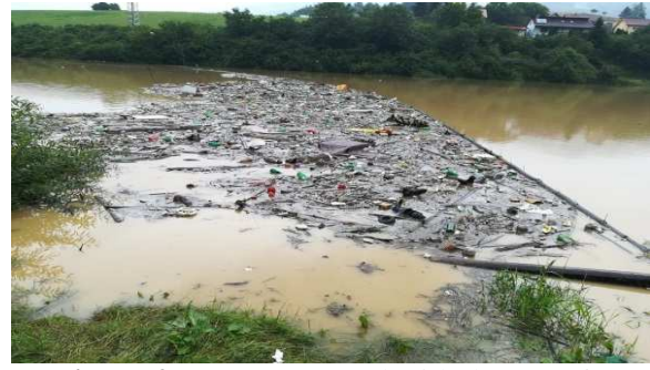
Figure 2. Waste captured with the use of a burrow wall in the area of the Ružín water reservoir Source: authors (2023)
