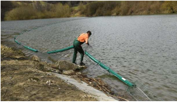
Figure 1. Installation of floating trash barriers in the area of the Ružín water reservoir Source: authors (2023)
