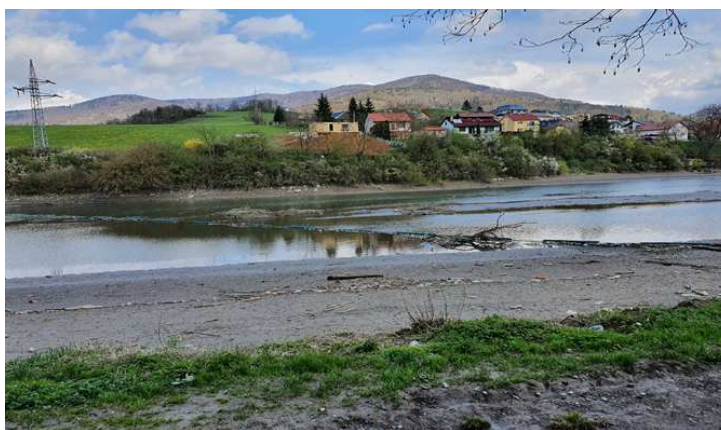
Figure 5. Installed floating trash barriers in the area of the Ružín water reservoir Source: authors (2023)
