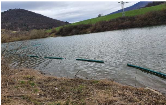
Figure 3. Installed floating trash barriers in the area of the Ružín water reservoir Source: authors (2023)
