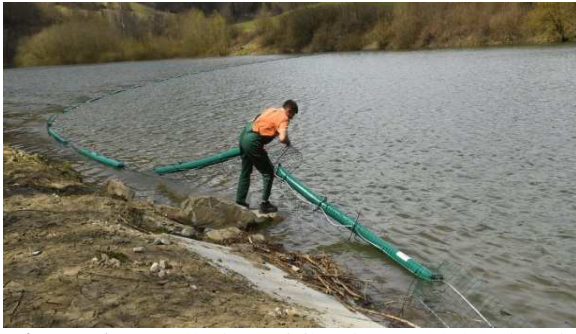
Figure 1. Installation of floating trash barriers in the area of the Ružín water reservoir Source: authors (2023)
