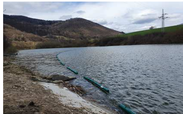
Figure 4. Installed floating trash barriers in the area of the Ružín water reservoir Source: authors (2023)
